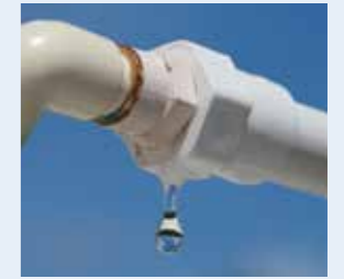
Leak detection in water pipes.
