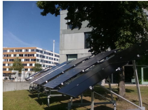
Figure 3.1: The set-up of the installed solar panels.
