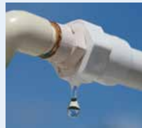
Leak detection in water pipes.
